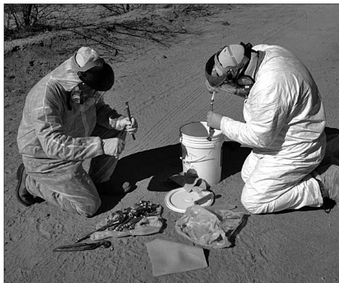
Bill, left, and Wes Reidhead add odorant to make the natural gas detectable.
