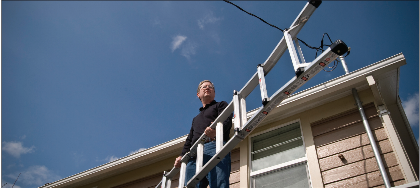
Ladders and power lines do not mix. Look up and around before any outdoor project. Note all of the potential safety hazards.
