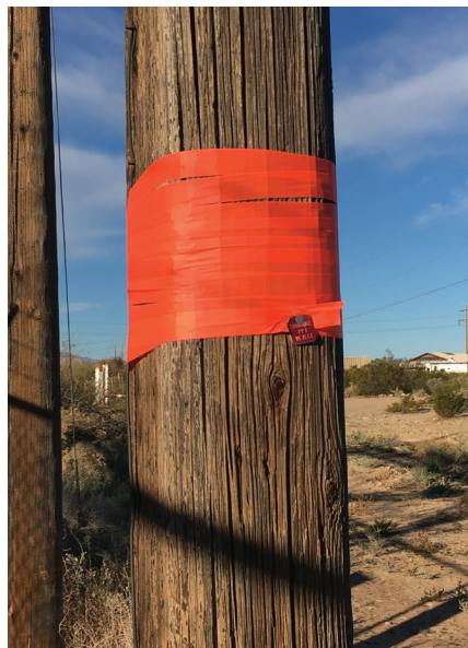
CLOCKWISE FROM TOP: A new line of poles is nearly ready to replace a stretch in need of repair. A damaged pole is marked for repair with orange flagging tape. A Sundance PPI crew member tests the base of a power pole for rot.
