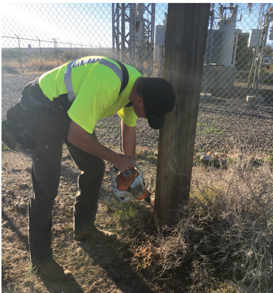
CLOCKWISE FROM TOP: A new line of poles is nearly ready to replace a stretch in need of repair. A damaged pole is marked for repair with orange flagging tape. A Sundance PPI crew member tests the base of a power pole for rot.
