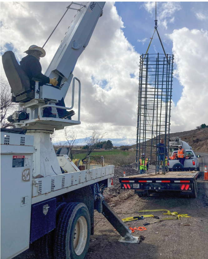
CLOCKWISE FROM ABOVE: Metal poles and wire span a section of the roadway. A rebar cage is readied for lowering into the hole to form the pole base. Crews pour concrete to create the stable base needed to anchor the metal power poles.
